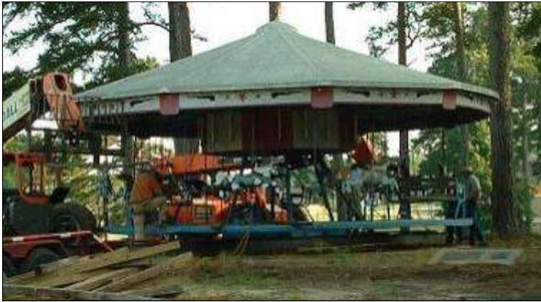
Workers preparing to lift the carousel for its move to the Depot Museum.
